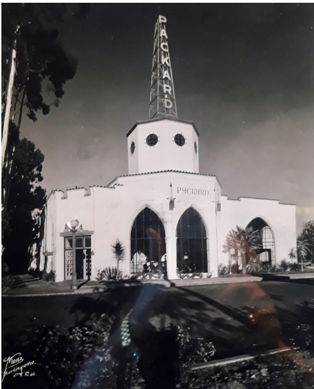
The Candy Store, shortly after it was built as the Packard dealer in 1928.
